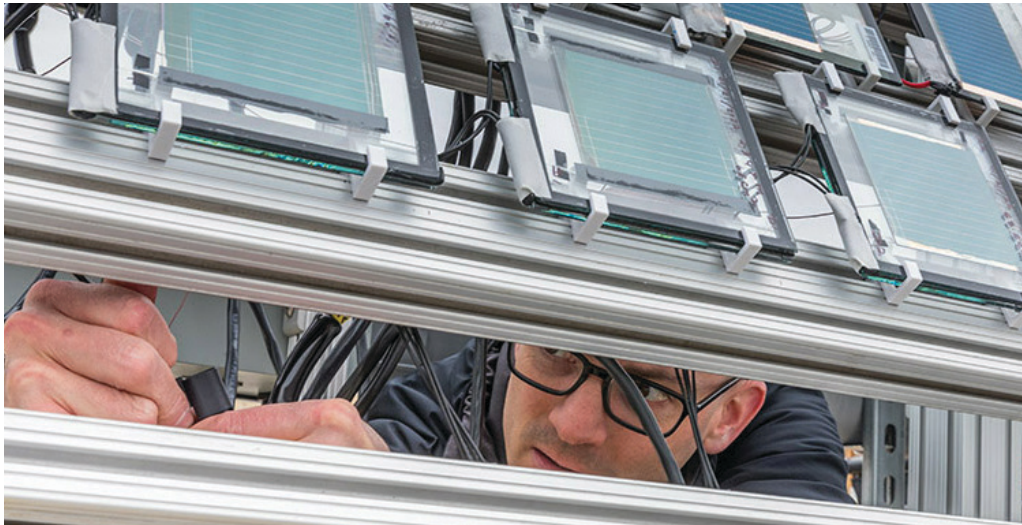
Photo by Werner Slocum, NREL.
